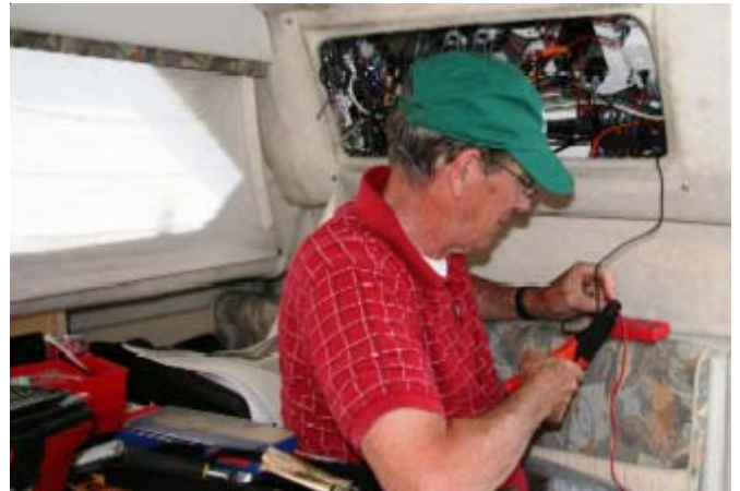
Harl Porter repairing the wiring on Walsh's boat Reely Fun .
