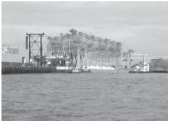
Detonation of the charges demolishing a 500-foot section of the Pearman Bridge.
